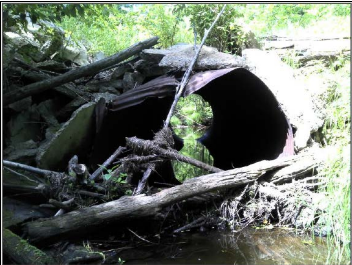
Figure 22. Road crossing on Perry Creek, downstream of assessment on 6/28/2016.
